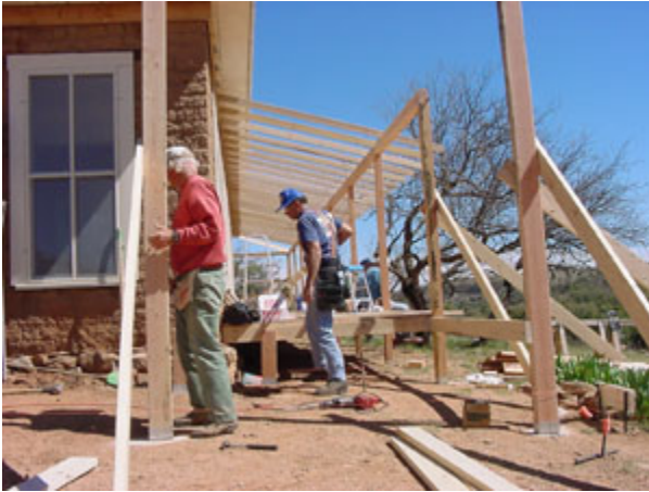
Steve Harper and Mark South framing the porch
