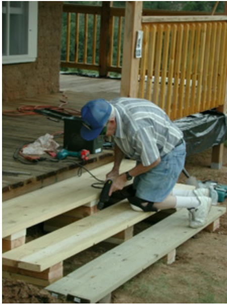
Jack working on porch steps
