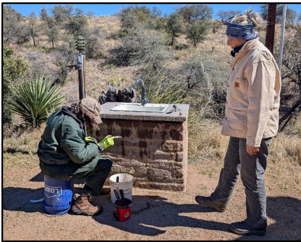
Susan Bierer and Gail Ryser putting on the finishing touches to the outdoor sink.
