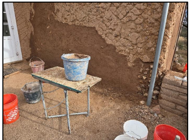
Spring caretakers Mark and Matt Doll did a fantastic job of applying a sacrificial adobe coat to the rental cabin.
