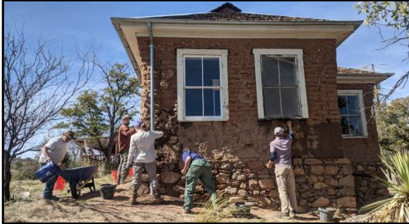
Sacrificial mud being applied to the southeast wall of the Gold Processing Building.
