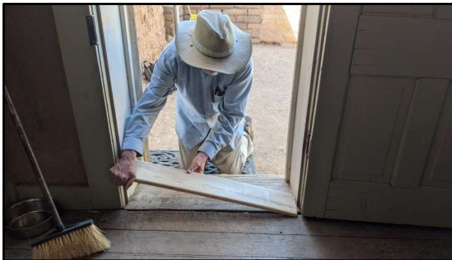
John Weiss fits a newly-crafted threshold board into a doorway.
