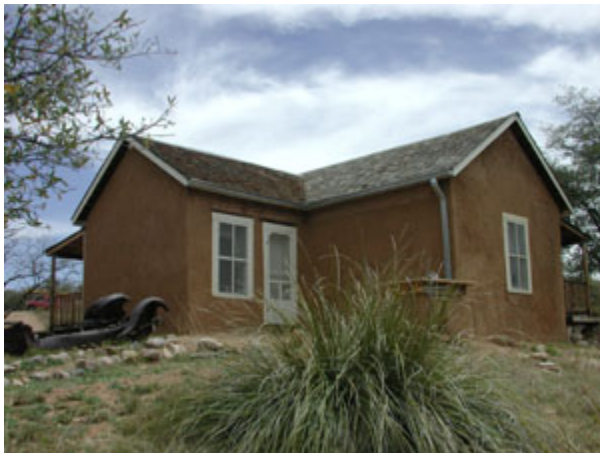
The outside walls of the Cabin are now beautifully finished.
