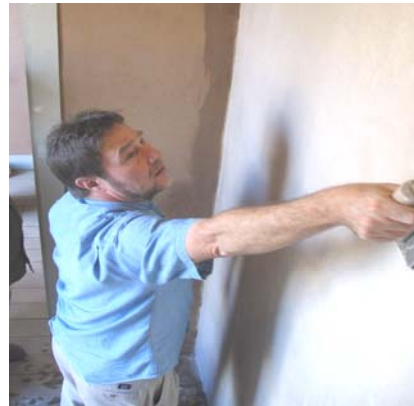
John Weiss applies texture to the kitchenette wall.
