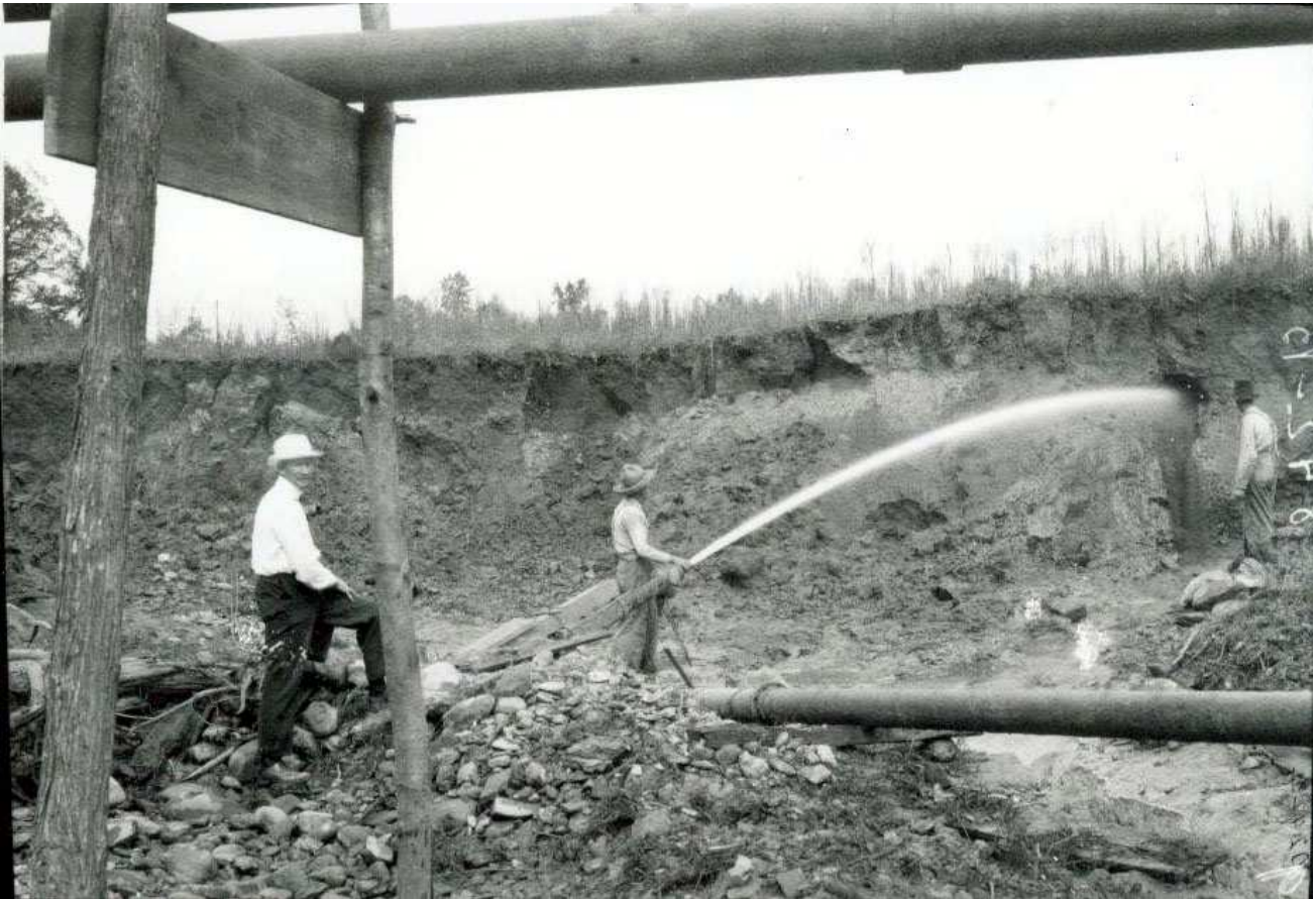
Yahoola River & Cane Creek Hydraulic Hose Mining Company - courtesy Georgia Dept of Archives and History (no known connection with Kentucky Camp or Santa Rita Water and Mining Company but similar equipment and techniques were used) For more information about the Yahoola River & and Cane Creek Hydraulic Hose Mining Company, aim your internet browser at: http://www.goldrushgallery.com/news/gordon.html
