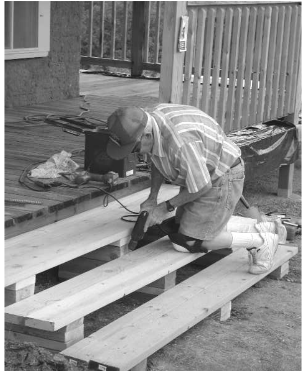
Jack Glenn building steps at Headquarters Building, 2001
