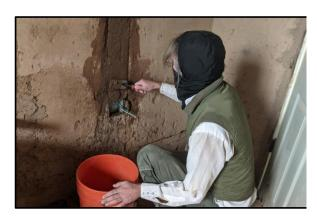
Last year's monsoon season resulted in some very heavy rains at Kentucky Camp. Some of this rain made it through the aging wood shake shingle roof and did some minor damage to the plastered and painted walls in the Blue Room. Thanks to Chris Schrager and his fine masonry skills, this damage has been repaired.
