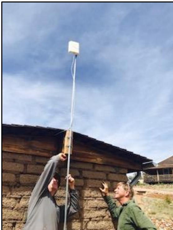
Ron Parrish adjusts the new cell phone booster antenna while Mark Doumas supervises. Photo courtesy of MarthaJo Billy
