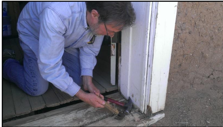
John Weiss prepares door threshold for new screen door. June 14, 2014 volunteer day. (Photo courtesy of Mark Doumas)
