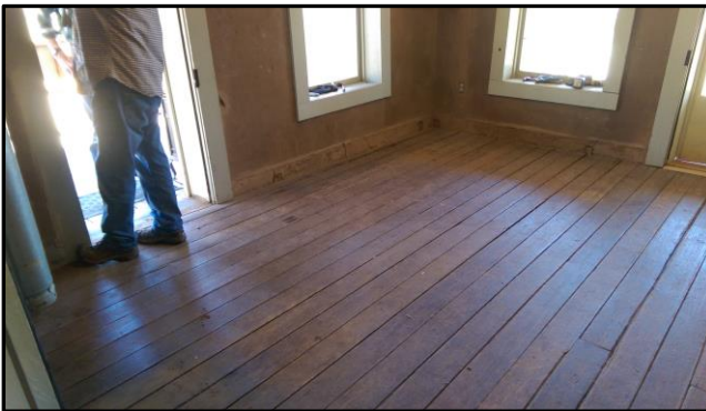
The end result: solid, good looking floors!
