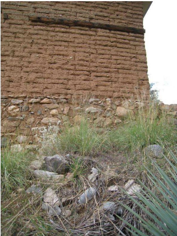
Chemical storage room corner stones and 2 x 4 roof attachment.
