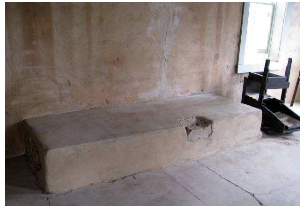
Concrete feature with two pipes at edge of the platform.
