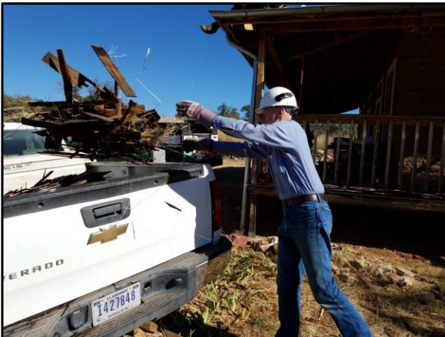
Pete van Cleve tosses away old shingles.
