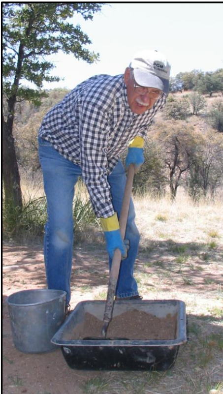
Jim Britton prepares mud plaster at the 2008 Kentucky Camp work week.
