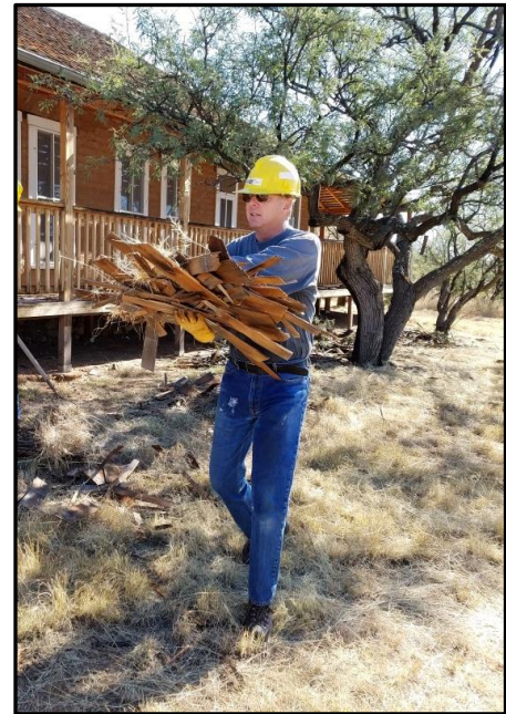
Ron Parrish cleans-up old shingles.
