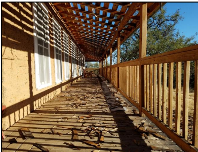
The Headquarters porch after removal of 16 year-old wooden shingles.
